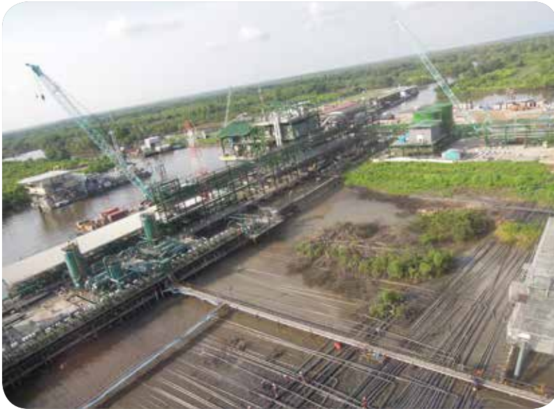
Upon extraction, the raw natural gas is saturated with water vapour and needs to be dehydrated
