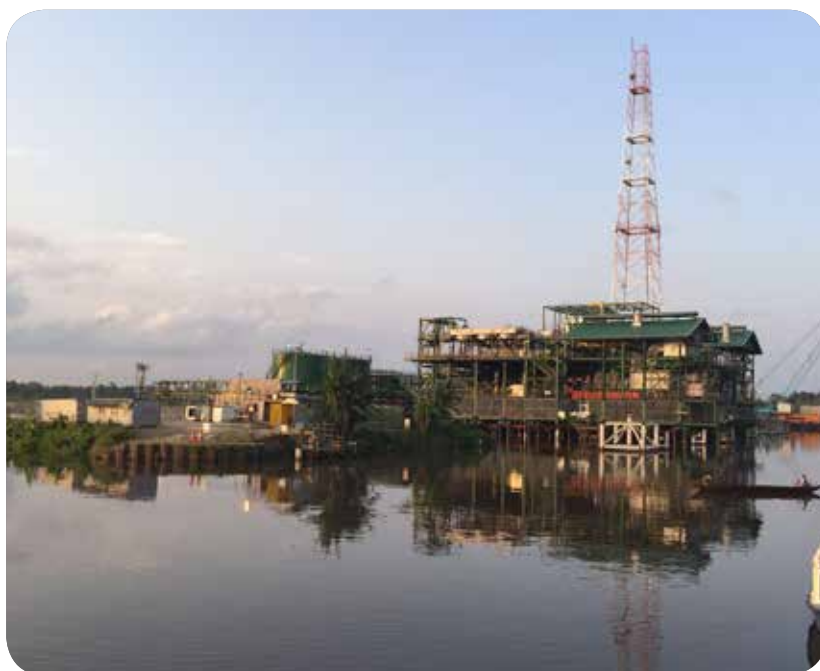
Gas dehydration, glycol regeneration and low-temperature separation at an extraction facility in Otumara, Nigeria
