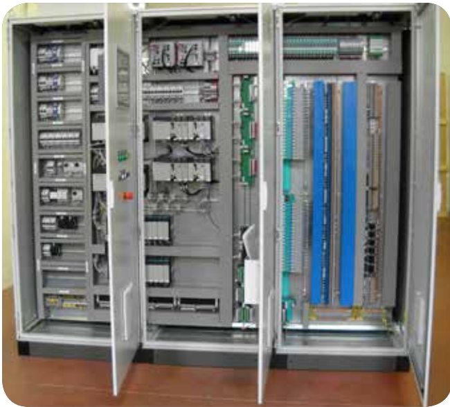
The end-customer imposed standardisation, which required a considerable evolution in the control system architecture
